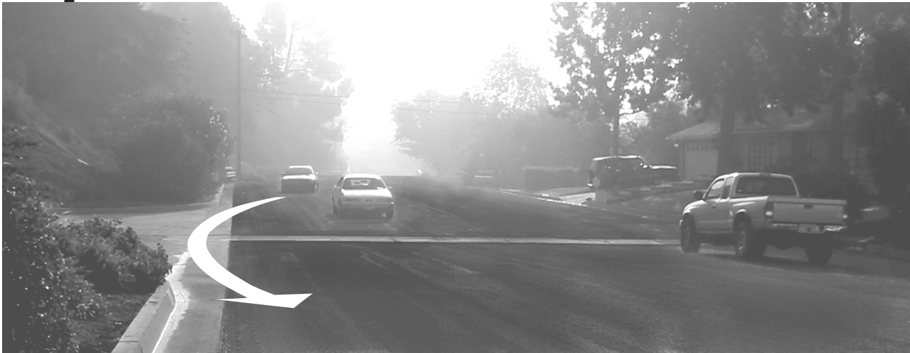
Intersection of Loma Alta and Stonehill Drive
